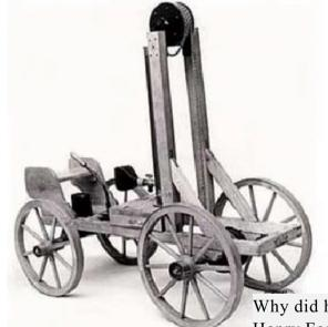
The first hydrogen car invented was not a fuel cell vehicle but rather an internal combustion engine. Swiss inventor Francois Isaac de Rivaz in 1807 designed the first 4-wheel prototype (pictured left) that ran on hydrogen and oxygen gas. The hydrogen gas was contained in a balloon and the ignition was an electrical Volta starter.
